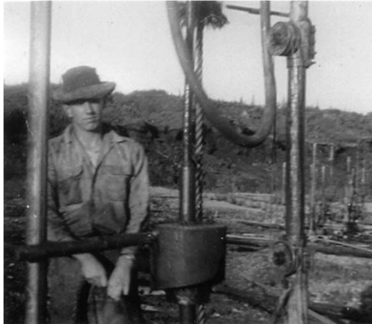
Dave Emerson Operating a Point Driving machine 1949
