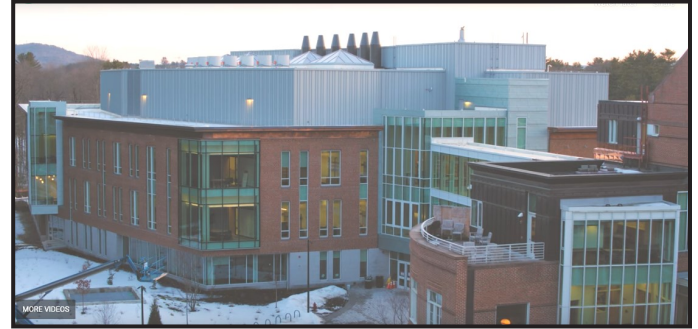
New Engineering and Computer Science Building
